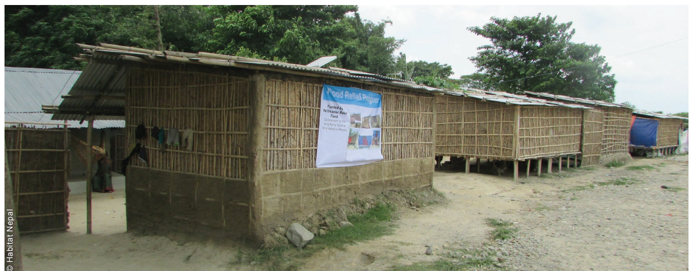
Shelters included mitigation features, such as raised floors, bracing and secure connections, and allowed for some adaptations, such as the upgrade of floors and walls.
