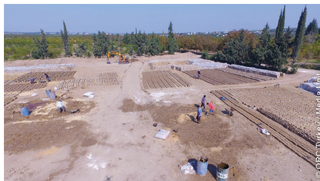
Adobe brick production required very large spaces and could only be conducted during the dry season. This caused some implementation challenges.
