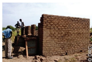
Mud bricks were mainly sourced from the local community, and partly through MoUs with landowners. Timber frames were prepared in workshops within the settlement.
