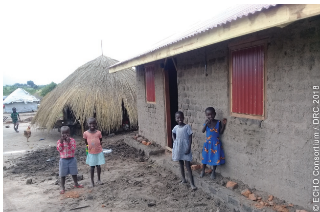
In Rhino the organization built larger, two-room shelters with CGI roofing.
