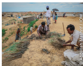
Site improvements were mainly conducted through cash for work and included slope protection by terracing (above-left) and vetiver plantation (above-right).
