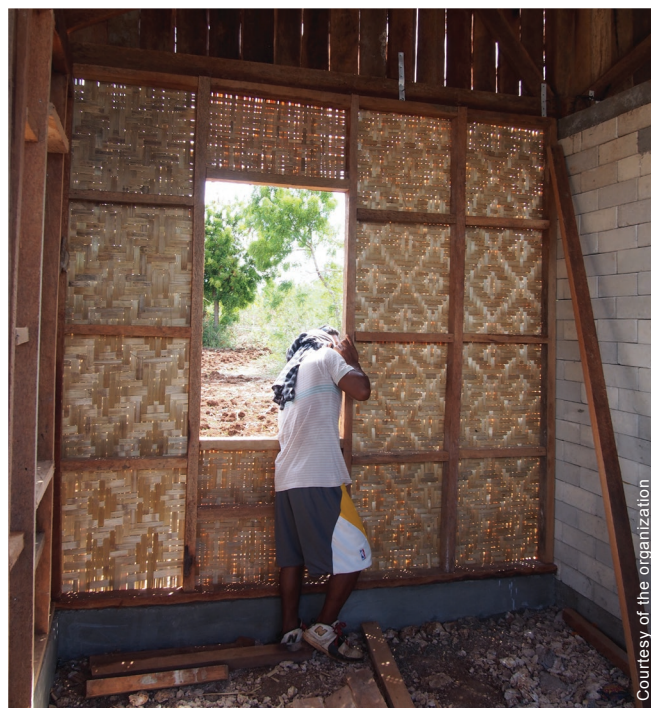
The adjoining room was made with a structure in coco lumber protected with a termite treatment, and an amakan walling. This could be replaced or re-design, so some families could built extensions for small kitchens and dining areas.
