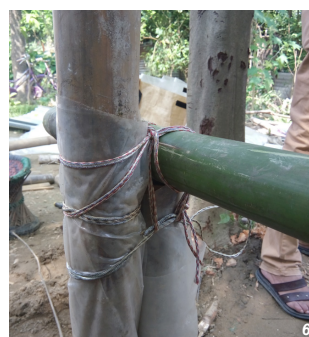
Left (4-5): Cut the required length of floor and roof posts with saw, tie them together and wrap them with polythene sheet. Cut the upper ends of the posts with a fish-mouth cut. Right (6-7): Place and tie floor beams to the bamboo floor post with rope. Place the next set of beams on top, perpendicular to the beam below. Place split bamboo joists above the floor beams. (Photo credits: Habitat Nepal).
