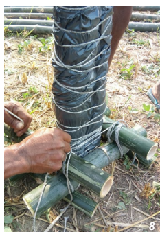
Left (8-9): Tie bamboo posts to the anchorage and place it inside the post hole. Then fill the hole with debris and tamp using wooden tamper. Right (10): Tie diagonal bracings of required dimensions to the roof post. Then tie the horizontal bracing at lintel level. Place the roof beams on top of the bamboo post and tie with rope. Place the cross bracings at roof level and then tie to the beams with rope. Right (11): Place bamboo purlins on top of the roof beam and tie with rope. Arrange 8 CGI sheets over them leaving one sheet width vacant in the middle. Tie 2 layers of purlins together to hold the CGI sheets in place. Place the remaining CGI sheet over the void and place 3' length purlins on top of each purlins below to hold the sheet down. This provides air movement inside the shelter through the roof. (Photo credits: Habitat Nepal).
