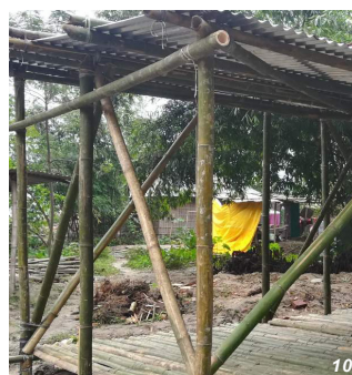
Left (8-9): Tie bamboo posts to the anchorage and place it inside the post hole. Then fill the hole with debris and tamp using wooden tamper. Right (10): Tie diagonal bracings of required dimensions to the roof post. Then tie the horizontal bracing at lintel level. Place the roof beams on top of the bamboo post and tie with rope. Place the cross bracings at roof level and then tie to the beams with rope. Right (11): Place bamboo purlins on top of the roof beam and tie with rope. Arrange 8 CGI sheets over them leaving one sheet width vacant in the middle. Tie 2 layers of purlins together to hold the CGI sheets in place. Place the remaining CGI sheet over the void and place 3' length purlins on top of each purlins below to hold the sheet down. This provides air movement inside the shelter through the roof. (Photo credits: Habitat Nepal).
