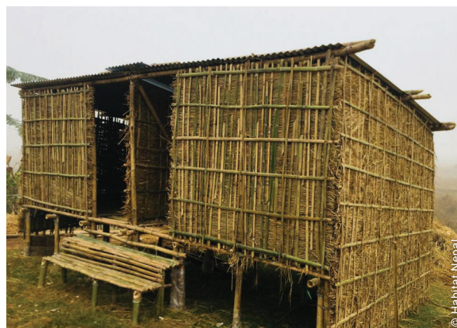
The project provided emergency shelters for flood-affected populations using local materials, and was implemented by local organizations who trained community members on bamboo construction techniques.
