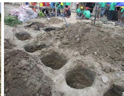
Left (1): Draw lines for foundation according to the dimensions and place the stakes in the ground. Check whether the stakes are at right angle using the 3-4-5 method. Centre and Right (2-3): Dig 21 post holes of 2' x 2' in the ground. (Photo credits: Habitat Nepal).
