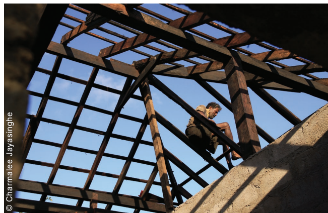
Roof work in progress in Vavuniya district. DRR features were included in roofs, foundations and walls. The gradient was increased to enable better run-off.
