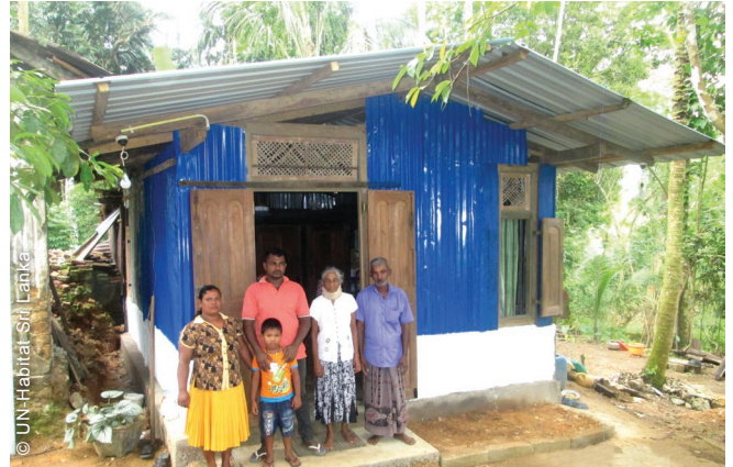
In some cases, transitional shelters were also built using salvaged materials.
