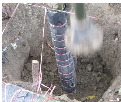
Left (8-9): Tie bamboo posts to the anchorage and place it inside the post hole. Then fill the hole with debris and tamp using wooden tamper. Right (10): Tie diagonal bracings of required dimensions to the roof post. Then tie the horizontal bracing at lintel level. Place the roof beams on top of the bamboo post and tie with rope. Place the cross bracings at roof level and then tie to the beams with rope. Right (11): Place bamboo purlins on top of the roof beam and tie with rope. Arrange 8 CGI sheets over them leaving one sheet width vacant in the middle. Tie 2 layers of purlins together to hold the CGI sheets in place. Place the remaining CGI sheet over the void and place 3' length purlins on top of each purlins below to hold the sheet down. This provides air movement inside the shelter through the roof. (Photo credits: Habitat Nepal).
