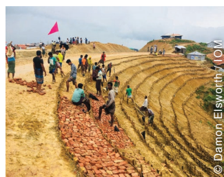
Site improvements were mainly conducted through cash for work and included slope protection by terracing (above-left) and vetiver plantation (above-right).
