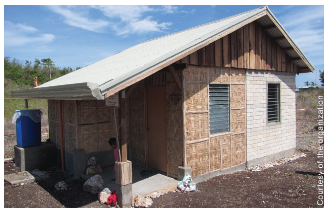
The project provided core houses with light-weight extensions, based on a common rural design. The houses included a gutter and a water tank for rainwater collection.
