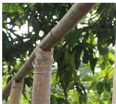
Left (4-5): Cut the required length of floor and roof posts with saw, tie them together and wrap them with polythene sheet. Cut the upper ends of the posts with a fish-mouth cut. Right (6-7): Place and tie floor beams to the bamboo floor post with rope. Place the next set of beams on top, perpendicular to the beam below. Place split bamboo joists above the floor beams. (Photo credits: Habitat Nepal).
