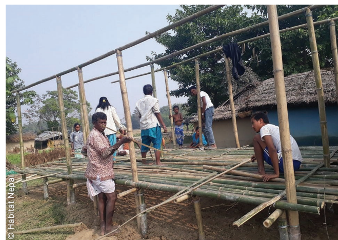
The project provided emergency shelters for flood-affected populations using local materials, and was implemented by local organizations who trained community members on bamboo construction techniques.
