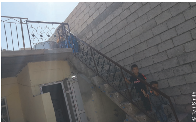
The project repaired walls and stairs, and added handrails for safety.
